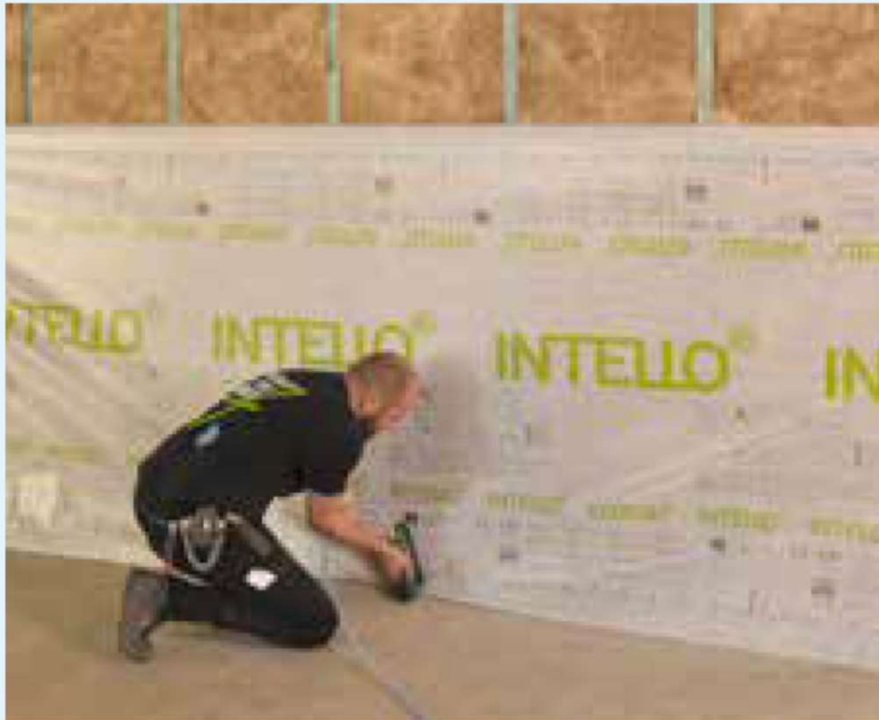
Figure 10.68: Installation of INTELLO® PLUS at wall sections
