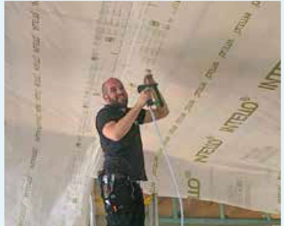
Figure 10.69: Stapling of INTELLO® PLUS. Photo courtesy of Bright Haus
