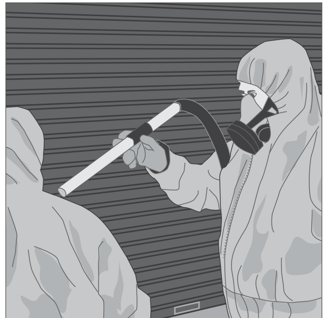
Figure 8: 'Buddy' cleaning – decontaminating colleagues with a Dust Class H vacuum cleaner.
