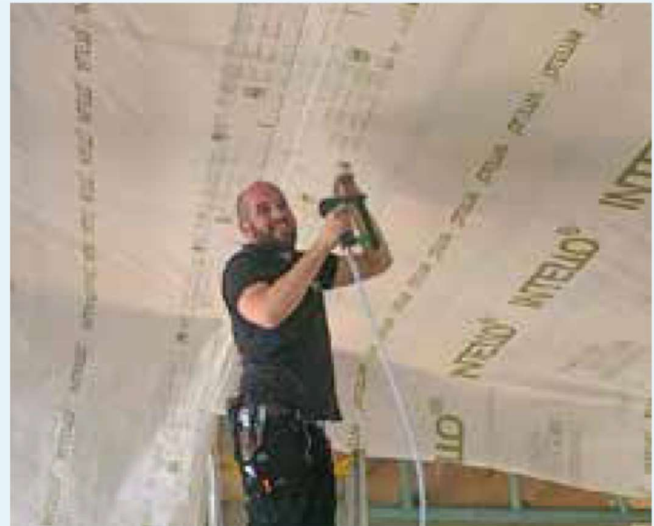
Figure 10.69: Stapling of INTELLO® PLUS. Photo courtesy of Bright Haus
