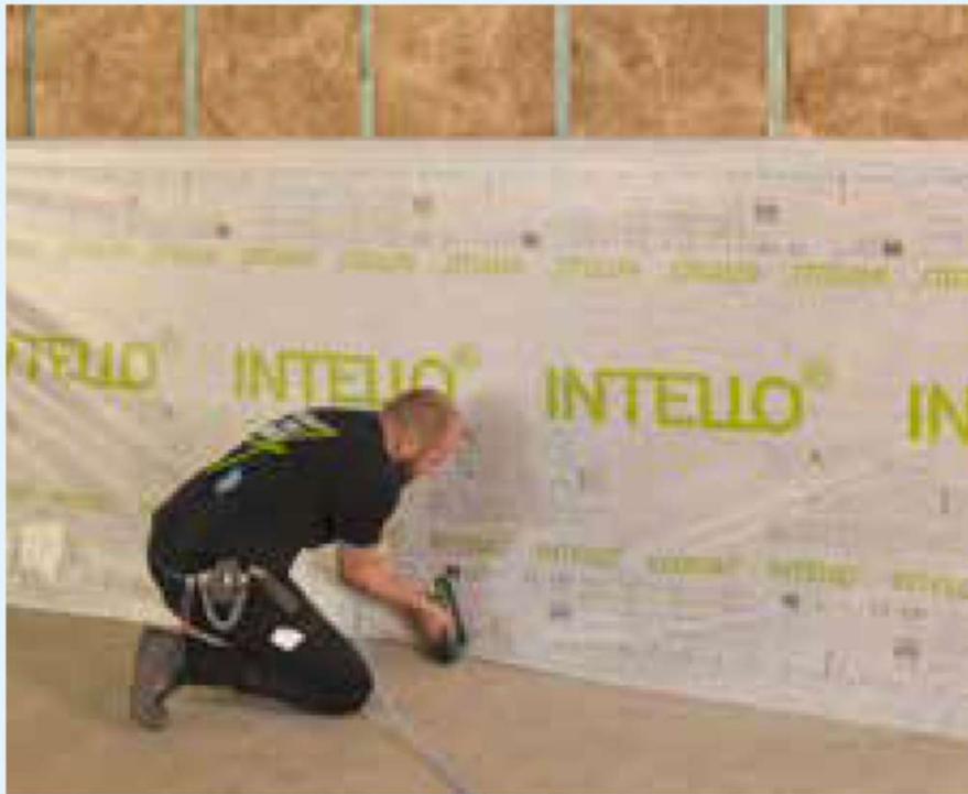
Figure 10.68: Installation of INTELLO® PLUS at wall sections
